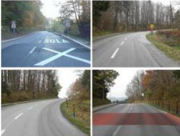
Figure 9: Improved road design in the vicinity of School and Kindergarten (direction "B")
